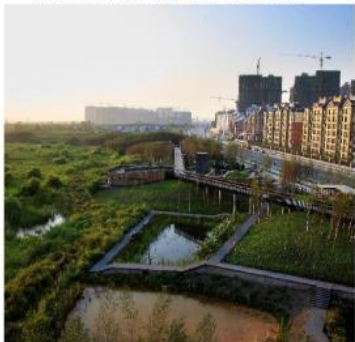
Qunli stormwater park te Harbin, China
